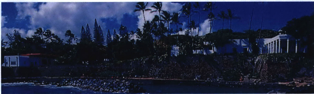
Fig. 13: Current elevation of Shangri La
