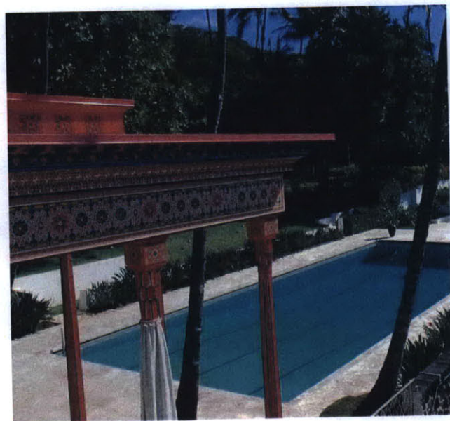
Fig. 22: Detail of roof and columns of Playhouse
